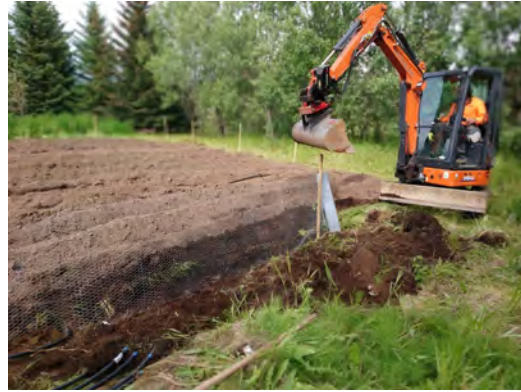
Figure 6: Setting the posts for the rabbit fencing.
