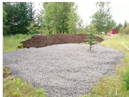
Figure 17: Already-present drainage gravel was spread before soil could be laid down.
