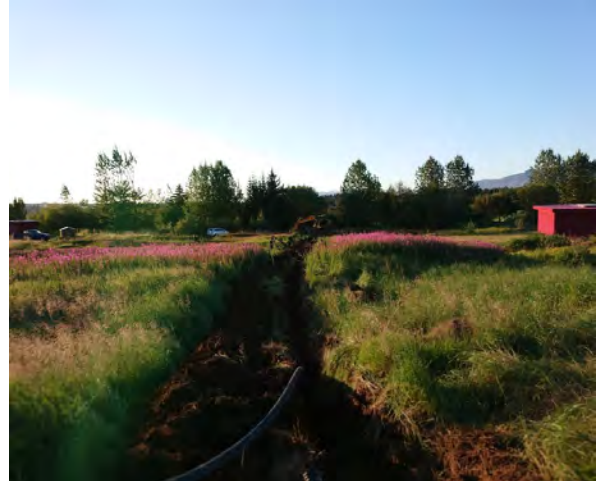
Figure 36: Insulated 25mm PEX from the source to the garden, being buried.
